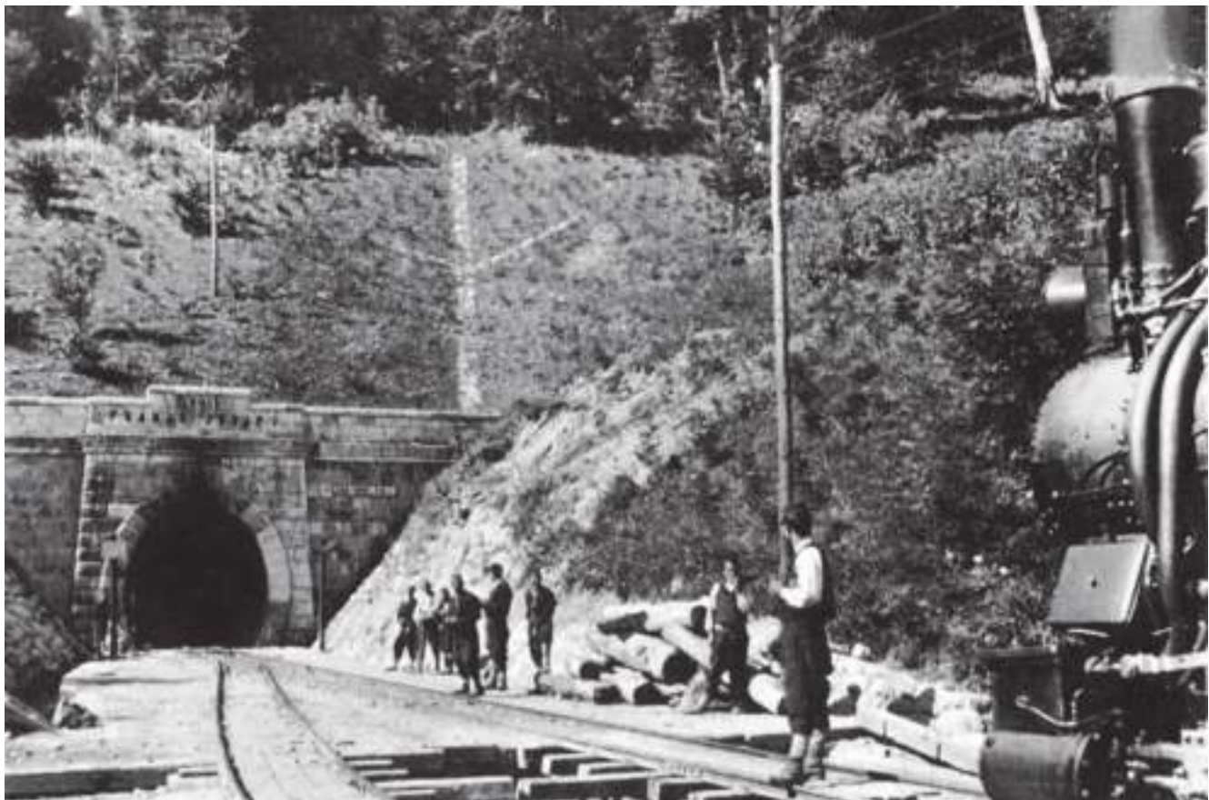
Slika br. 129: Željeznička stanica i tunel Ivan 1907/1908.
